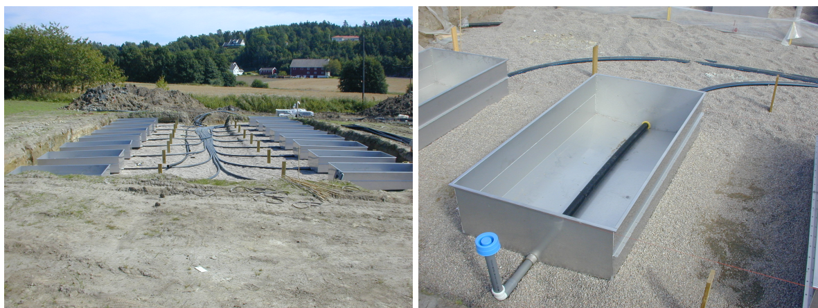
Photo 1 a,b. Lysimeters at construction in 2003. Photos: Trygve S. Aamlid.
