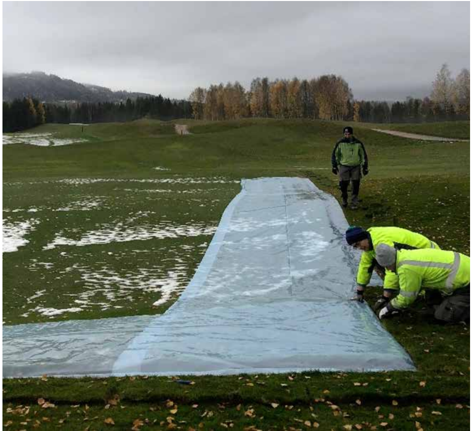
Photo 5. An important preparation is to dig plastic collars into the higher surrounds outside the green. In this case, the spring tarp and the impermeable cover can be fastened under the collar to prevent melting water from seeping in under the covers. Photo: Mads Thers.
