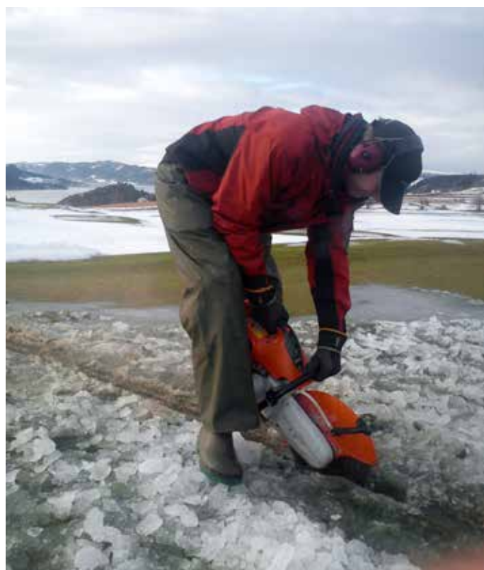
Photo 23. Temporary ditches in greens need maintenance during the winter. An asphalt cutter in use. Photo: Ole Albert Kjosnes, Byneset GC, Norway.
